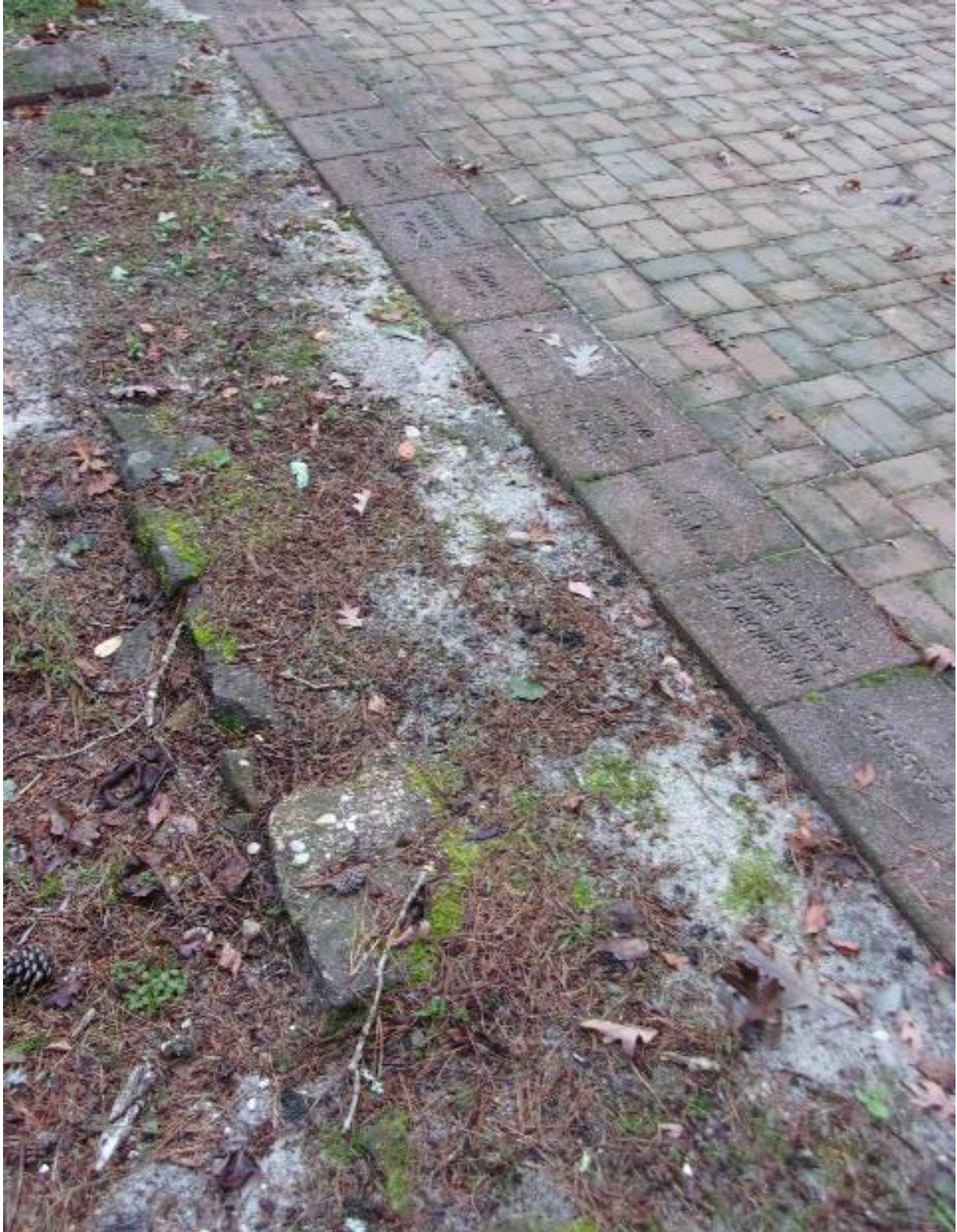
Plate 3-7 Remaining portions of the original ironstone foundation for the St. Mary's in the Pines church.
